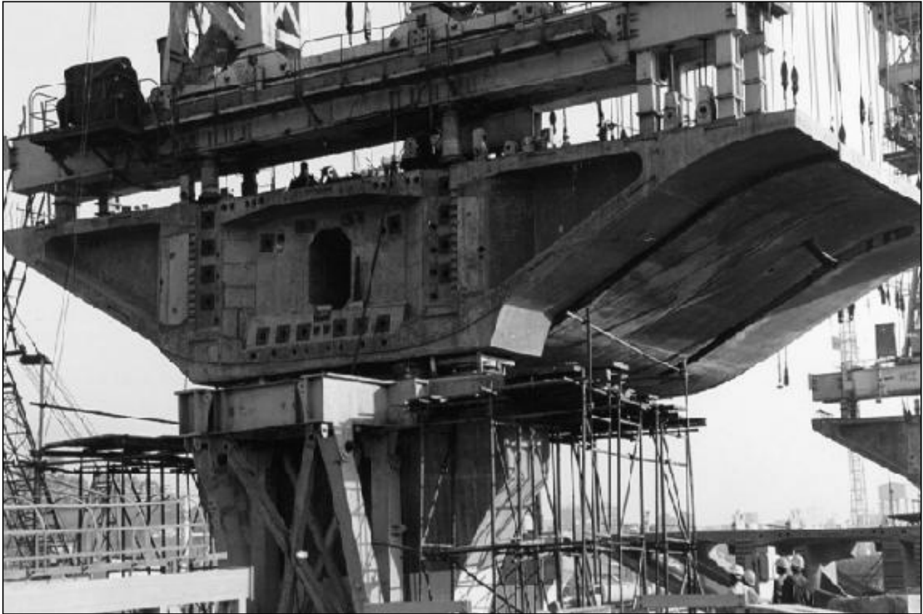
Figure 5. Erection of bridge segment over disc bearing in Bandra Worli Sea Link
