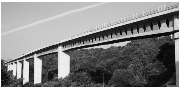
Figure 1. Butterfly Web Bridge
