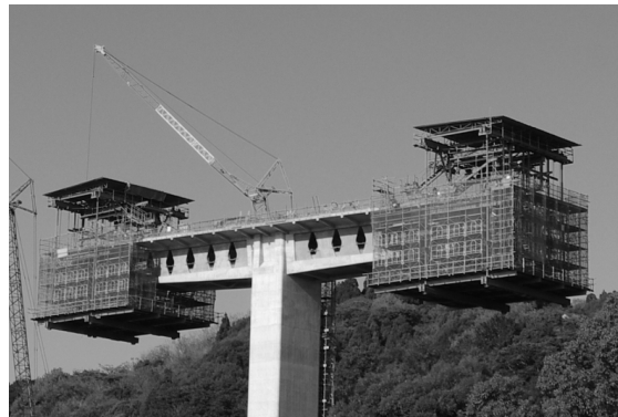
Figure 13. Cantilever construction
