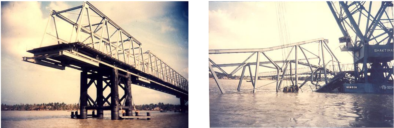
(a) (b) Figure 9. Image of bridge after the collapse (a) Part of Karnaphuli bridge (looking towards south), (b) Image of collapsed span along with the crane that hit the bridge. The undamaged part of the bridge is visible in the back.
