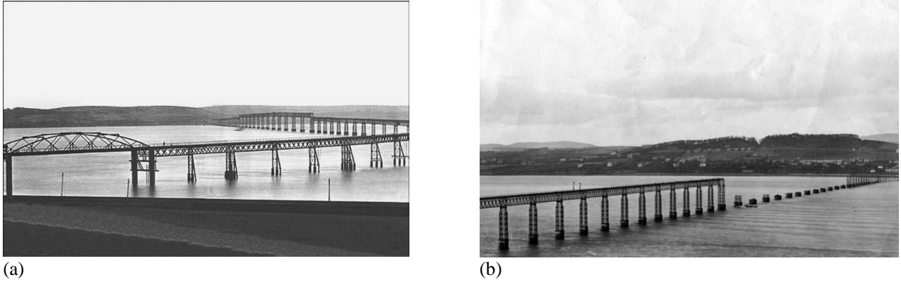
Figure 2. Images of Tay bridge, (a) Tay bridge just after completion in 1878, (b) Collapsed high girder section of the bridge with twelve pier platforms almost completely swept off from their high girders (Lewis and Reynolds 2002).
