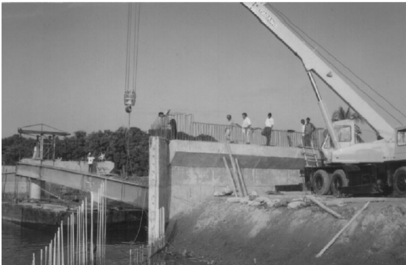
Figure 27. Construction of one of the initially selected 25 bridges
