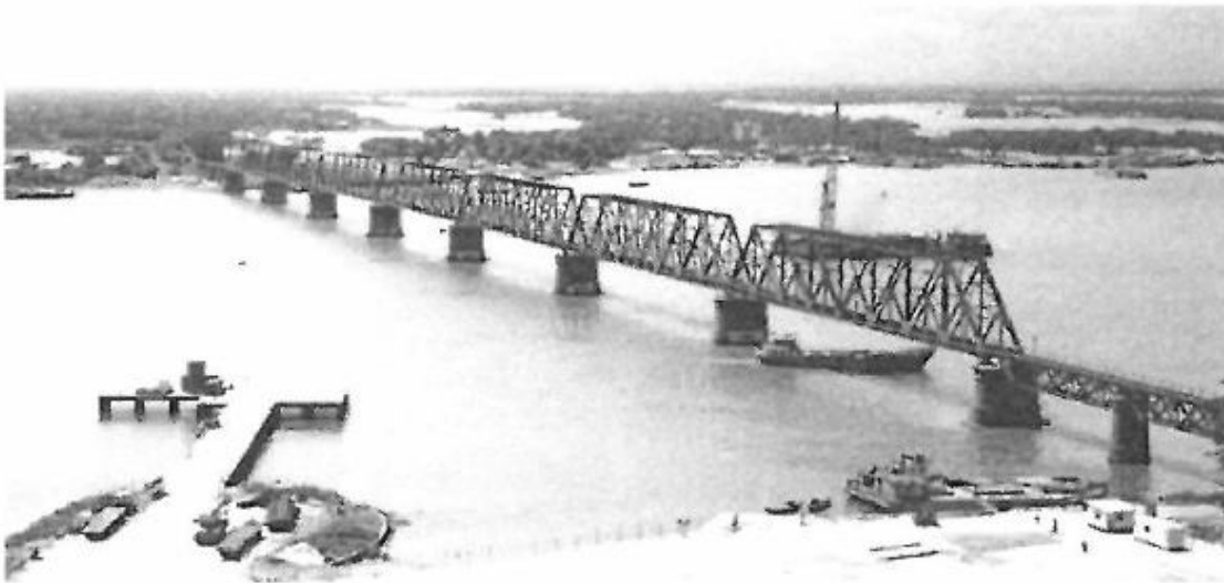
Figure 11. Bhairab Rail Bridge across the Meghna River
