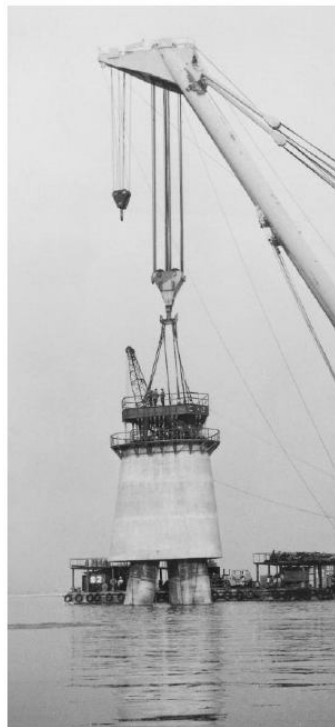
Figure 20. Placing a pile cap
