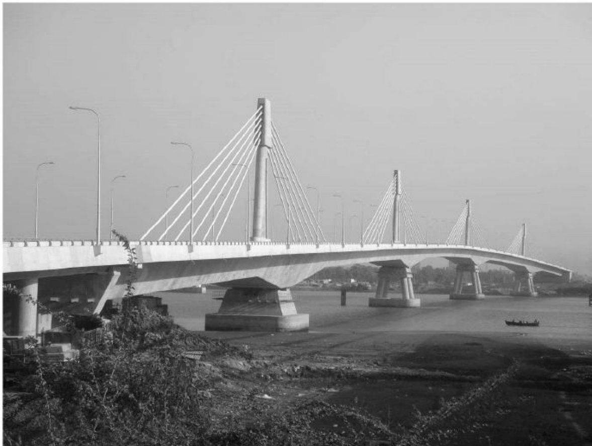
Figure 30. The Shah Amanat Bridge across the Karnaphuli River at Chittagong
