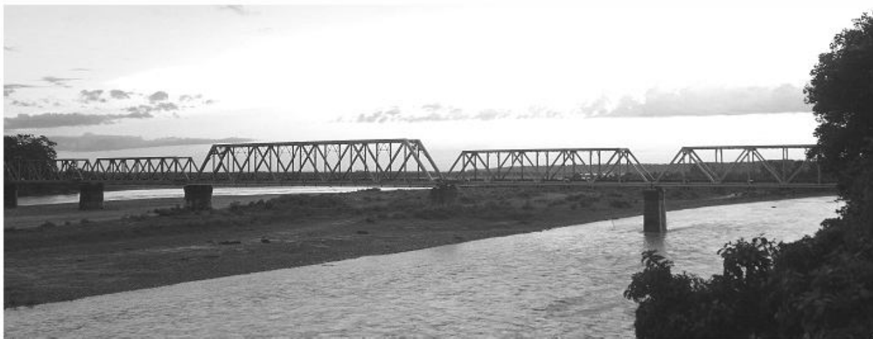
Figure 12. Sir Alexander Rendel's 1901 rail bridge across the Teesta river
