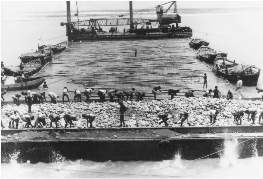
Figure 24. Floating out fascine mattress and sinking by ballasting with boulders
