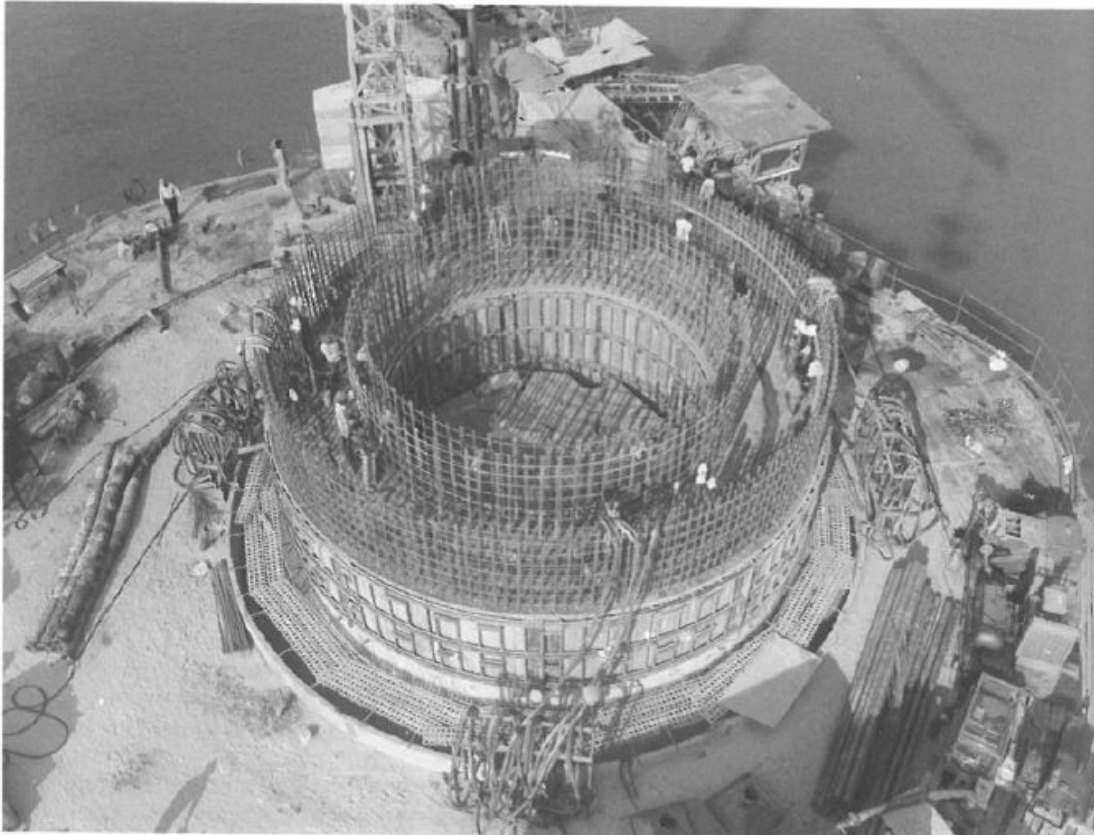
Figure 16. Caisson in sand island during sinking
