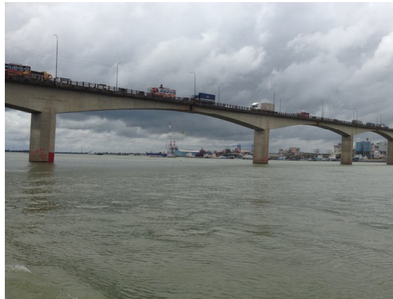
Figure 2. Meghna Bridge showing central hinge at the mid-span between Pier 9 and Pier 8 (marked in red)
