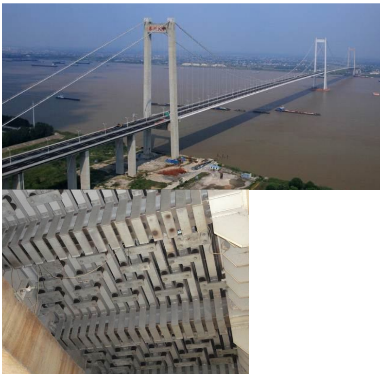
Figure 6. The new Taizhou Yangtze River Bridge (left) and a modular expansion joint on the bridge, viewed from below (right).
