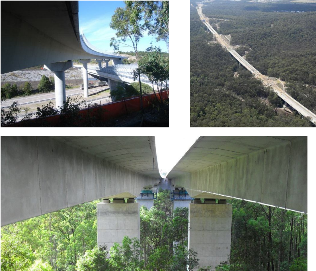
Figure 12. Views of various monitored structures of the Hunter Expressway.
