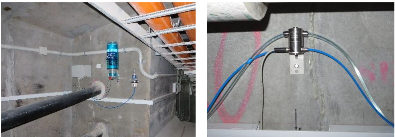
Figure 13. Installation of the monitoring system inside the concrete box girders of the Hunter Expressway.
