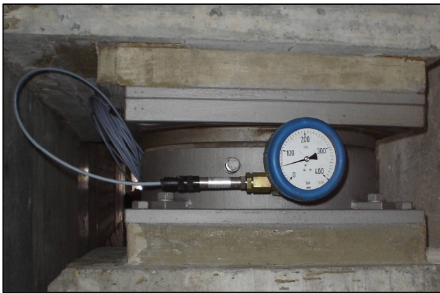
Figure 4. The ongoing condition of the Pont Nanin structure in the Swiss Alps has been monitored by an SHM system (with force monitoring at bearings as shown) since its static design was changed a decade ago (fixing at end).
