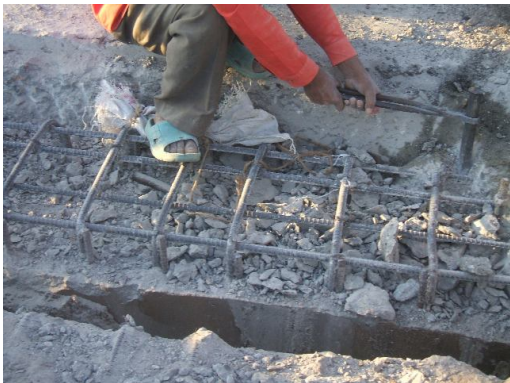
c) Chipping of concrete
