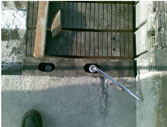
Installation of EJ & fixing of bolts
