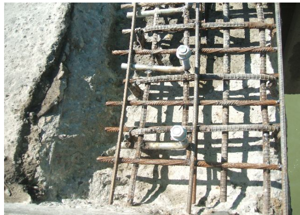
b) Additional bar reinforcement
