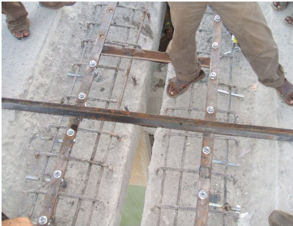
c) Setting of anchor bolts/templates
