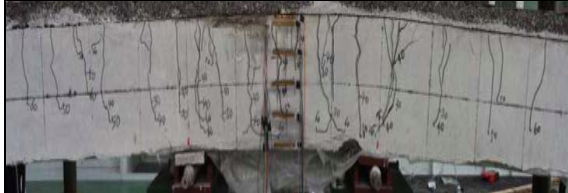
Figure 9. Damaged beam without CFRP
