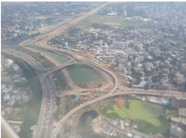
Figure 9. Panoramic view of constructed interchange
