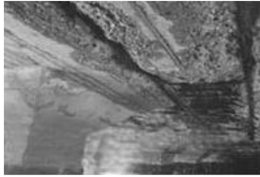
Figure 10. (a), (b) Reinforced concrete girders extremely damaged by corrosive environment
