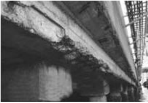
Figure 10. (a), (b) Reinforced concrete girders extremely damaged by corrosive environment
