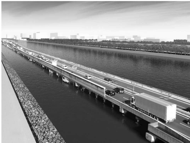
Figure 11. Current situation (before renovation)
