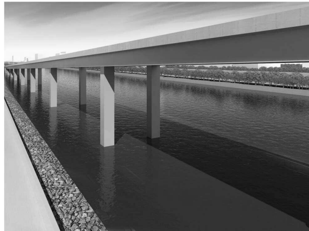
Figure 12. Viaduct after renovation
