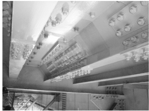
Figure 14. Reinforcement of orthotropic steel deck
