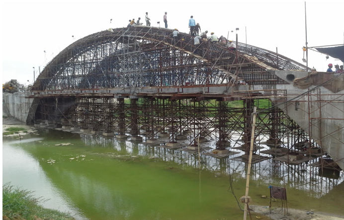
Figure 13. Photograph of scaffolding system and formwork of the bridge
