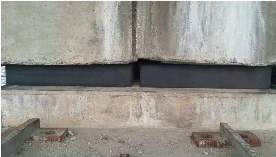
Figure 9. Photograph of replaced bearings
