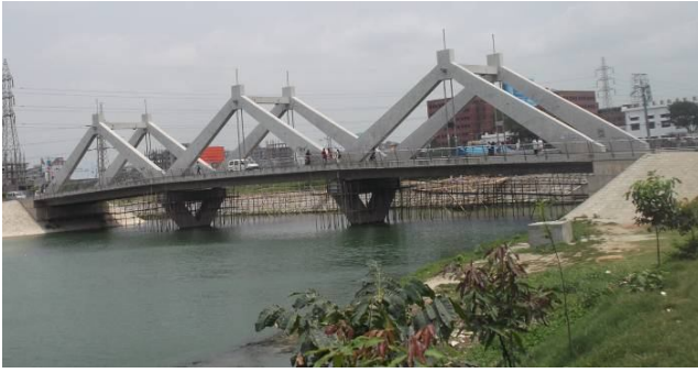
a) Photograph of the bridge
