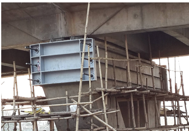
Figure 5. Retrofitted pier head
