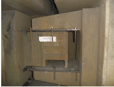
Figure 2. Failed attempt to stop slipping out of packing due to deck vibration.
