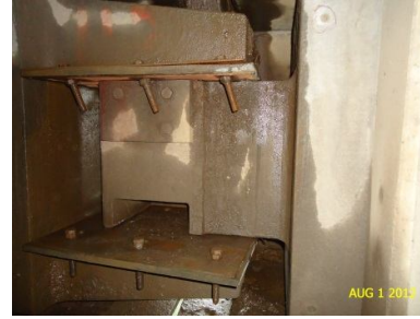
Figure 2. Failed attempt to stop slipping out of packing due to deck vibration.
