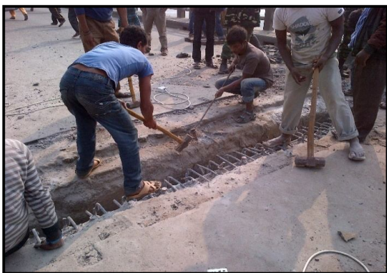
Figure 13. Hacking of concrete box-out.
