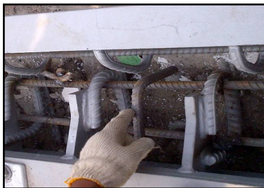
Figure 14. Finger joint installation in obstructive starter bars.
