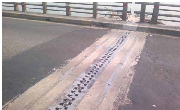
Figure 16. Installed finger joint.
