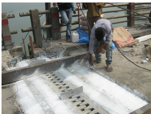
Figure 15. Application of curing compound after casting.
