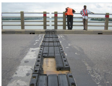
Figure 3. Expansion joint before rehabilitation.
