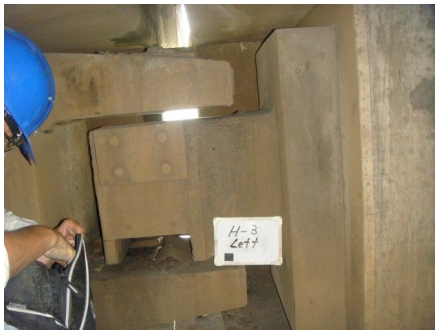
a) Gap before packing
