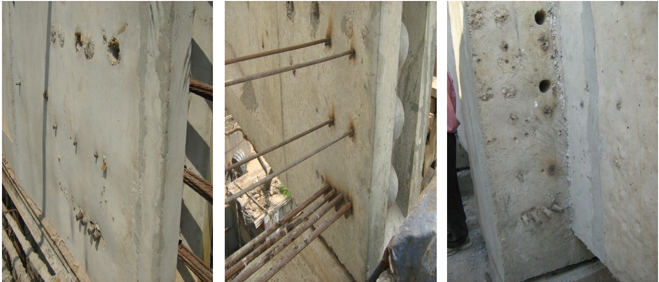
a) Continuity bars shaved off b) Inadequate lap of diaphragm bars c) Misaligned diaphragm
