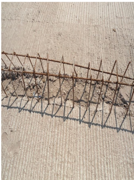
Figure 5. Poor riding surface of deck
