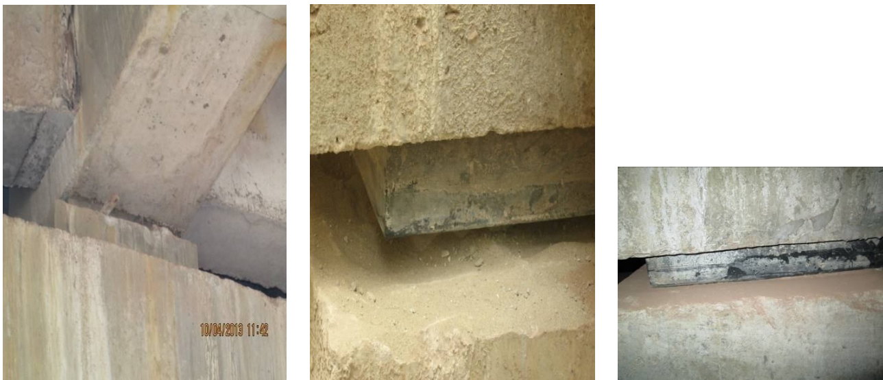
a) Bamboo packing under bearing pad
