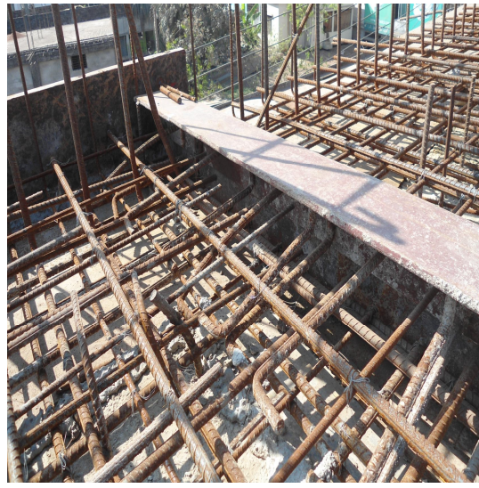
b) Makeshift edge beam with inadequate anchorage
