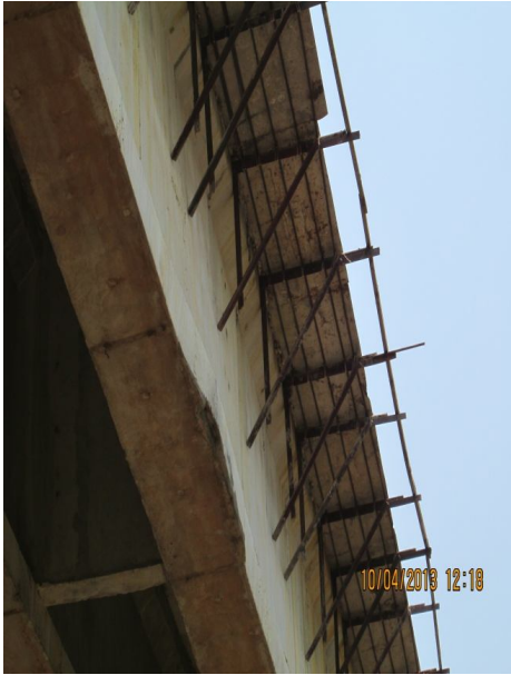
Figure 3. Bulging of girder concrete due to poor formwork
