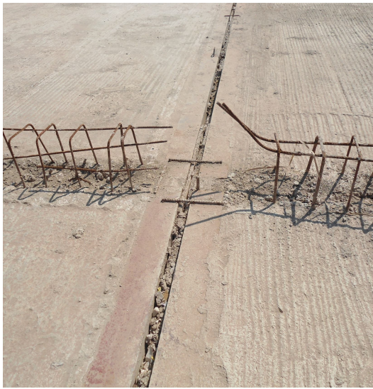
a) Installed expansion joint
