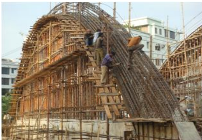
Figure 13. Banani bridge construction stage photograph of arch
