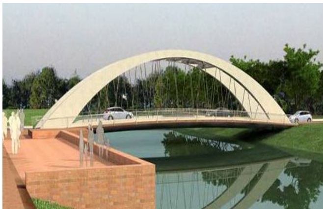
Figure 11. Arch bridge over Modhumati river at Gopalganj (Nielsen Type)
