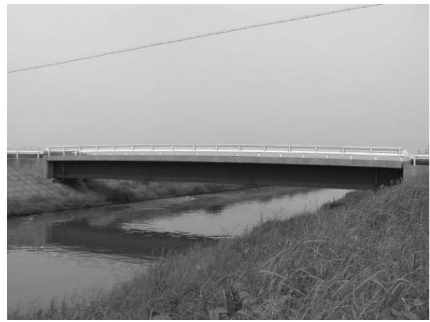
Photo 1. Overview of the bridge
