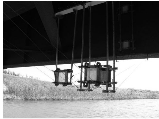
(b) Accumulator under the bridge
