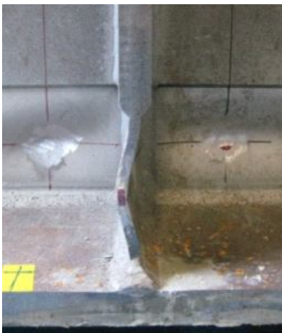
Figure 2. Local Buckling at Vertical Stiffener
