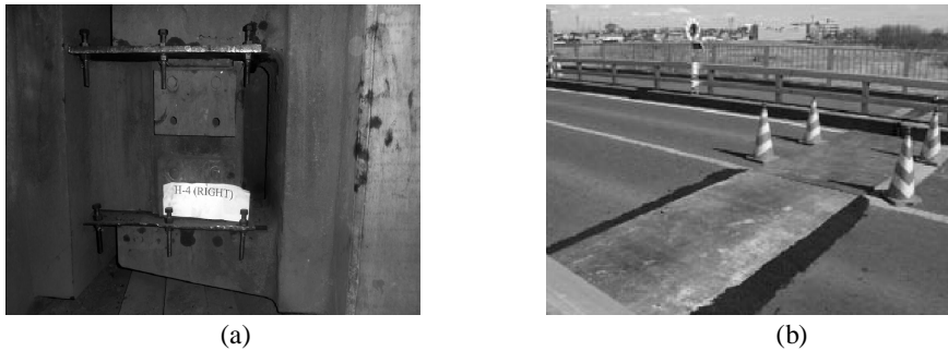
Figure 3. Repairing work of Meghna Bridge (a) steel plates were inserted at hinge location as a short term repair, (b) expansion joints were covered by steel plates at temporary repairing stage.
