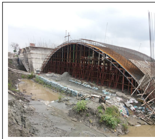
View of Arch & Abutment
