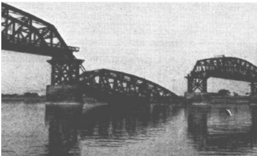
Figure 7. Fallen Span 12
