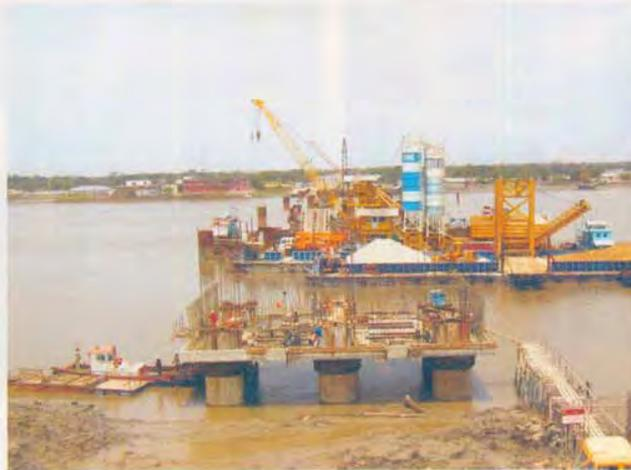
*In order to construct pile cap below the water level the precast concrete shell forms were constructed and hanged around the steel casing for main piles above the water level*
