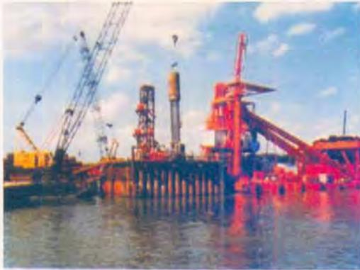
*Insertion of Steel Bar Cage inside Bored Pile*
