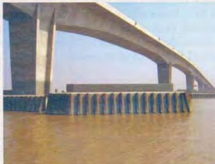
*Timber Fenders on Precast Fender Units*
