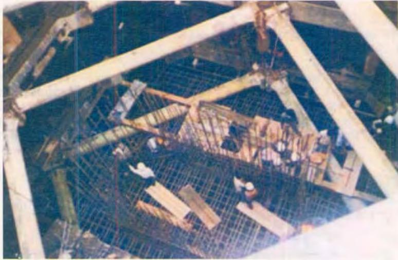
*Fabrication of Steel Bar in Pile Cap*
