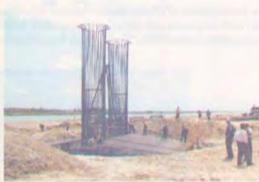
Re-bar Basing of Pile Cap and Pier Column Substructure
