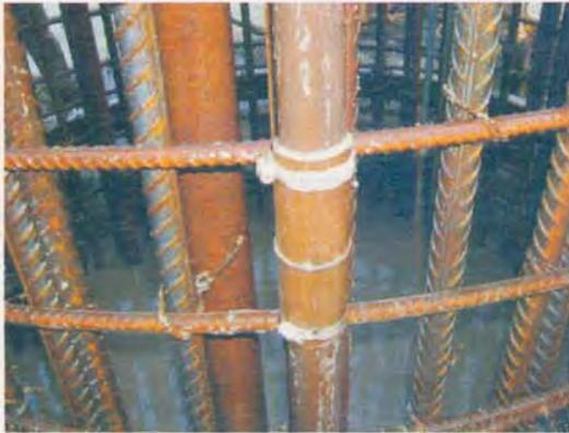
Grout Pipes Attached with Reinforcement Cage
