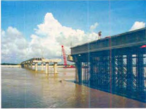
*Staging Formwork for Casting Deck and Girder*
