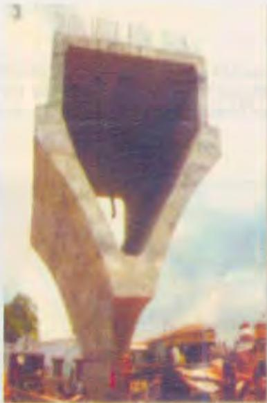
*Y-frame Constructed in-situ for Supporting 44m Long PC Girders*
