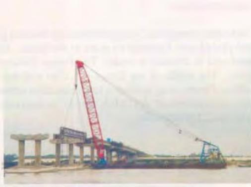
*Lifting of Launching of Girder*
