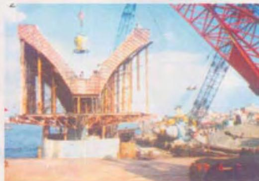
*Concreting of Y-frame of Pier*
