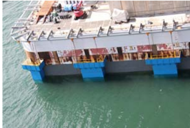
Photo 5. Protection work by “Dry Box”
