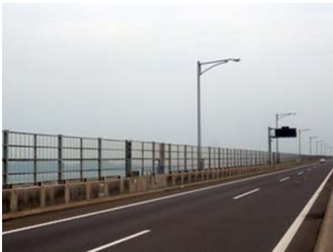
Photo 8. Windbreak fence on approach viaduct
