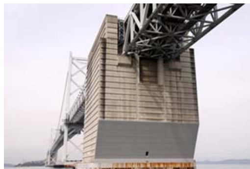
Photo 1. Anchorage of the Minami Bisan-Seto Bridge
