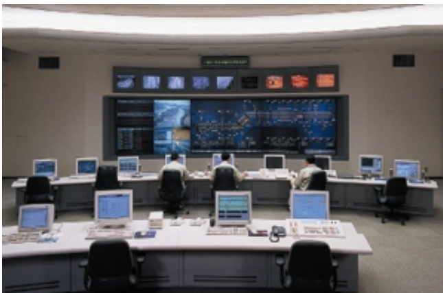
Photo 6. Graphic panel at traffic control center
