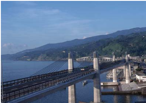
Figure 12. Odawara Blue Way Bridge (3-span continuous extradosed PC bridge)
