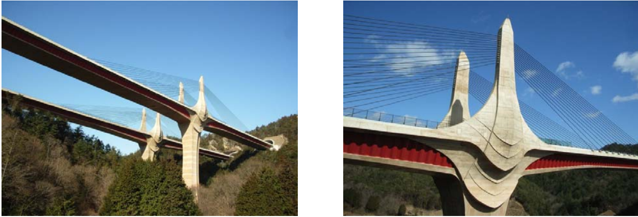
Figure. 21 Rittoh Bridge (Extradosed PC bridge with corrugated steel web)
