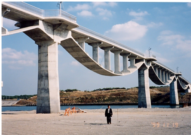
Figure 20. Shiosai Bridge (4-span continuous stress-ribbon PC bridge)
