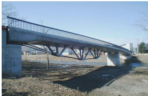
Figure 7. View of the completed Boukei Bridge
