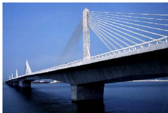
Figure 17. Ibi River Bridge
