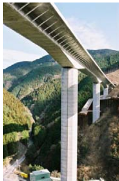
Figure 18. Shibakawa Viaduct (Continuous PC box girder with inclined struts)
