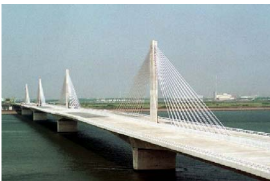
Figure 16. Kiso River Bridge
