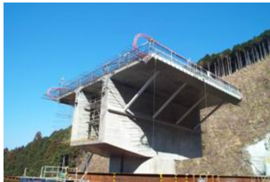
Figure 19. PC box girder with inclined struts
