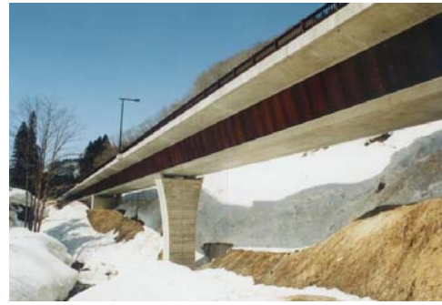
Figure 15. Ginzanmiyuki Bridge with corrugated web using atmospheric corrosion resisting steel
