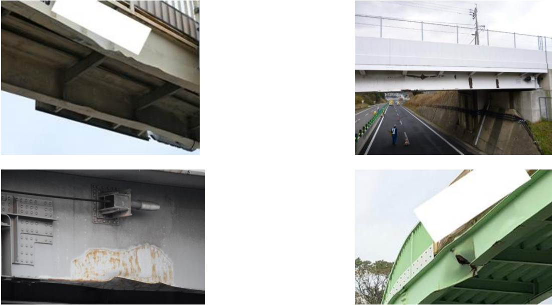
Figure 1. Bridges damaged by collision.
