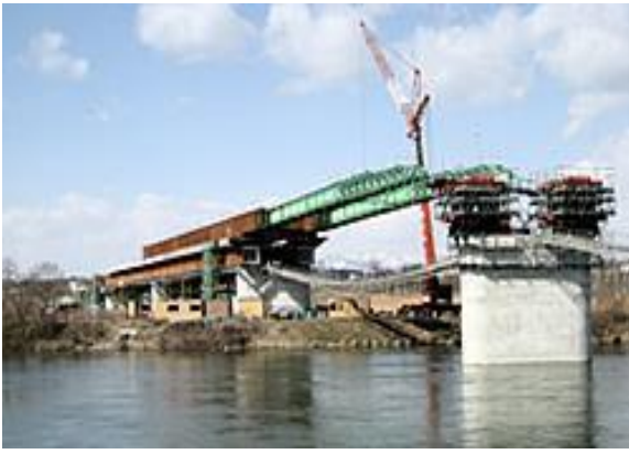
Figure 7. Use of nose girder for narrow box girder erection.
