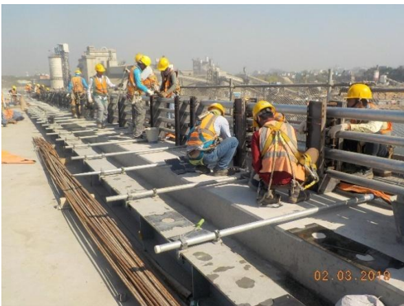
Figure 5. Use of PPEs by the workers during superstructure construction.
