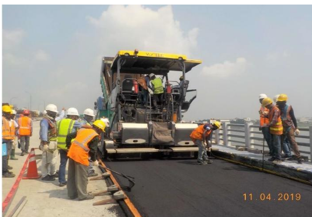
Figure 6. Use of modern road paving equipment and light drilling machine during road works.
