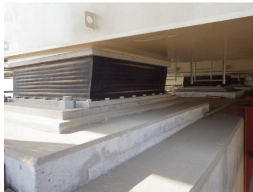
(b) High Damping rubber bearings installed in the 2 nd Meghna Bridge
