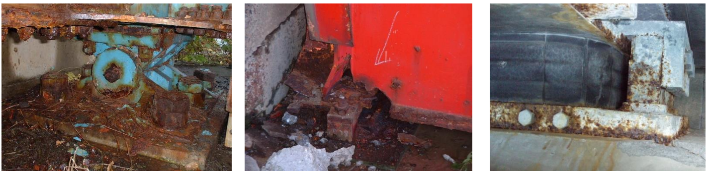
Figure 1. Corrosion of bridge bearings
