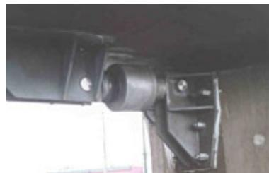
Fig. 18. STU between the substructure and the deck
