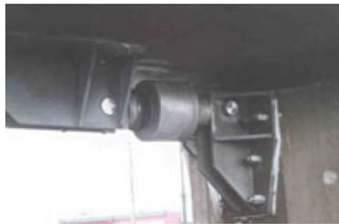
Fig. 18. STU between the substructure and the deck
