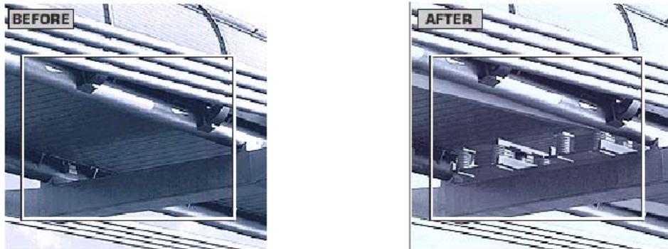
Fig. 3. Addition of tuned mass dampers in The Millennium Bridge
